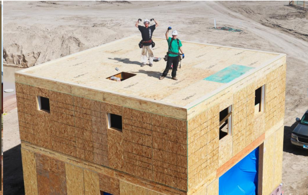
Thunder Valley CDC, Workforce Development, Porcupine, SD Sustainable construction
